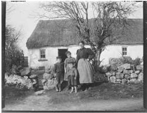
Open fire; insulation rare
