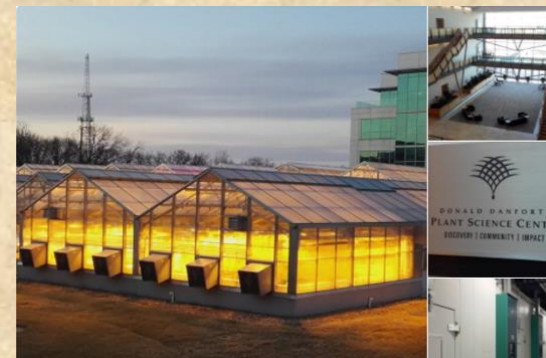
Extensive facilities at Danforth Center glasshouses, St Louis, Missouri
