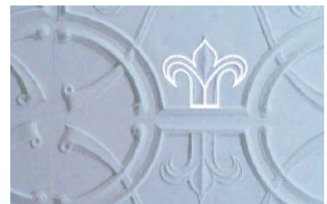
Plasterwork on the ceiling of the entrance hall of Brookfield House
