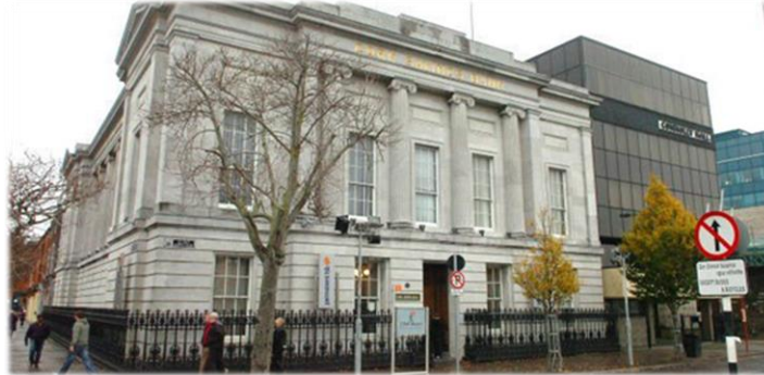
The Lapp's Quay Executive Education building currently under refurbishment.
