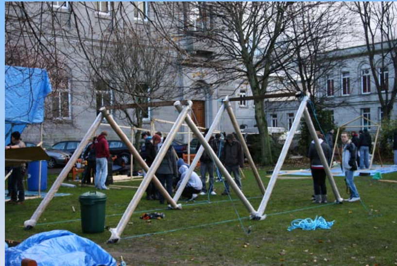
'The Cardboard Cradle', a design which incorporated recycled cardboard tubes from cardboard manufacturers
