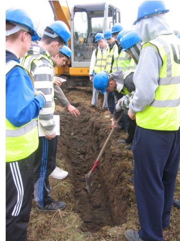
Figure 2 Trial pitting for geotechnical PBL
