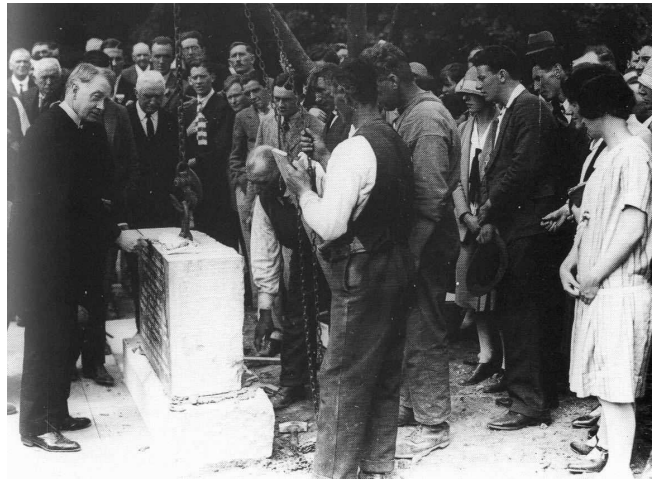
President Cosgrave lays the foundation stone for the Dairy Science building.
