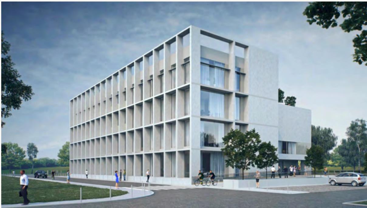
The Health Innovation Hub , due to be the first building in the Cork Science & Innovation Park at Curraheen, is currently being tendered by Buildings Contractors. Construction is expected to commence in Spring 2019.
