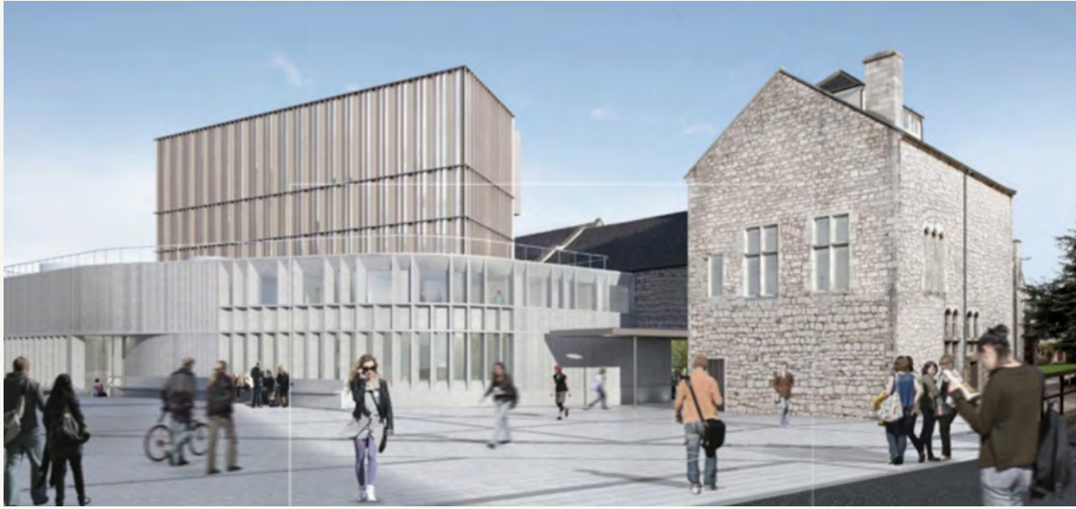
Work on the Student Hub is progressing well, expected completion in early 2019.
