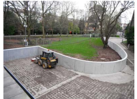
Flood Protection Glucksman
