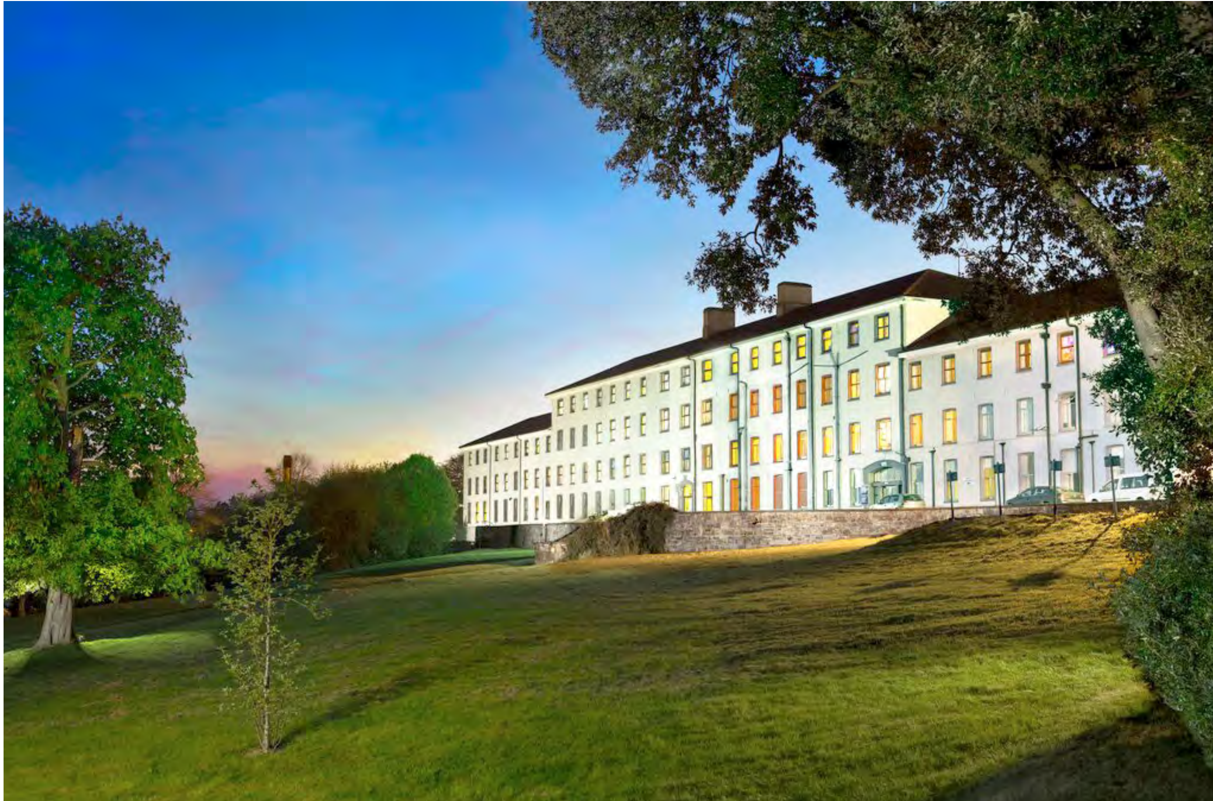
South Tipperary General Hospital
