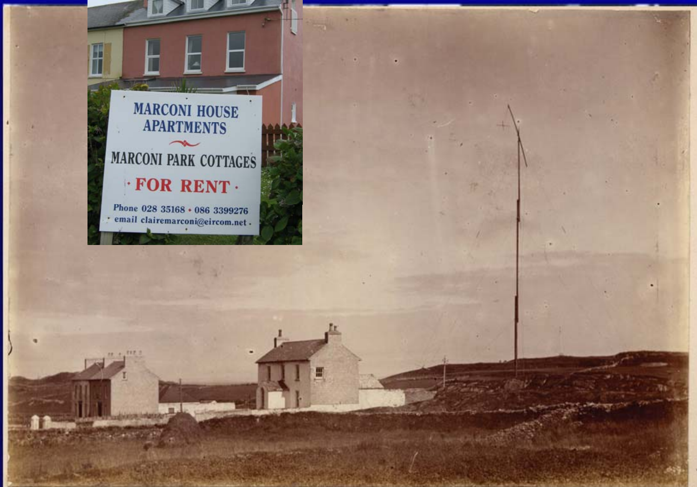
Marconi Station, Crookhaven. Co. Cork.
